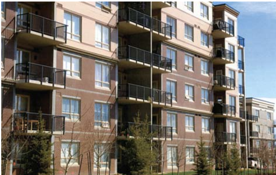
The Eagle Ridge condominiums in Fort McMurray, AB, Canada, satisfied skeptics of precast concrete’s aesthetics with its brick patterns, staining, and stucco design. Courtesy of Tucker Photography.
